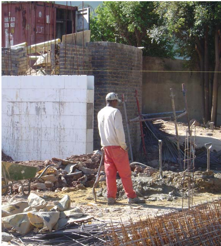
VARIBLOCK WALL UNDER CONSTRUCTION
