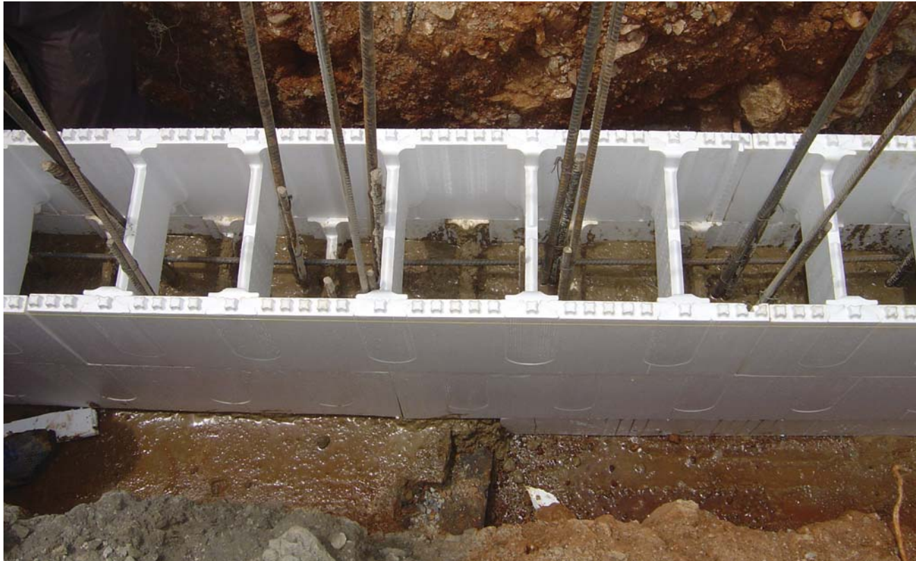
VARIBLOCK WALL UNDER CONSTRUCTION
