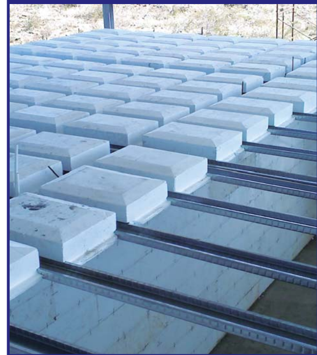
TASS installation in progress
